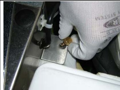
6 Remove the bin cover holding screws
